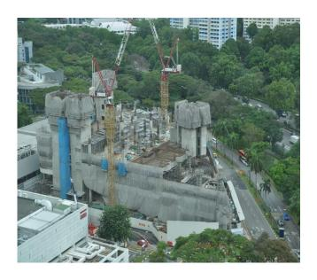
The main contractor for the construction of the National University Centre for Oral Health, Singapore (NUCOHS) commenced work on 1 February 2016. Significant construction activities in 2016 included the completion of piling and excavation works and the erection of the megatruss to cover NUH's existing cooling systems. As you pass by the site today, you would have probably seen a pair of tower cranes, the lift corewalls and the building superstructure from ground level to the 3rd storey.
